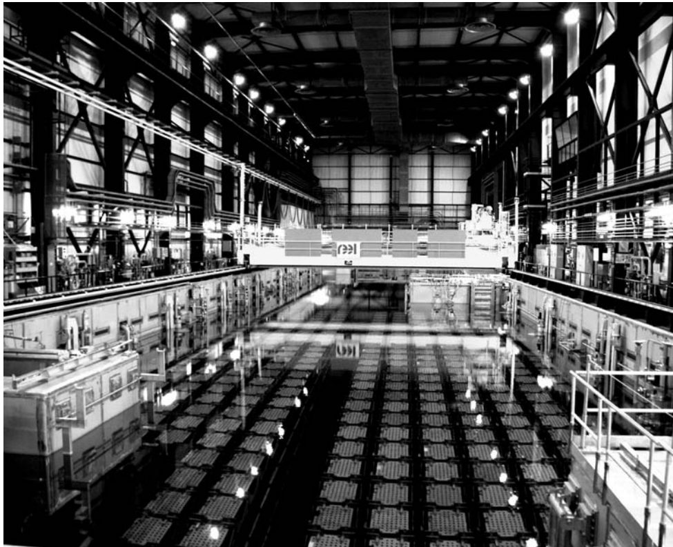
Figure 12.3. Clusters of dense-packed spent fuel in La Hague pool, 2012. Source: Sortir du nucléaire .
