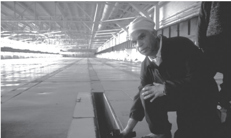
Figure 7.2: Technician looking under the cover over the huge storage pool for VVER-1000 spent fuel at the Mining and Chemical Combine in Zheleznogorsk.
