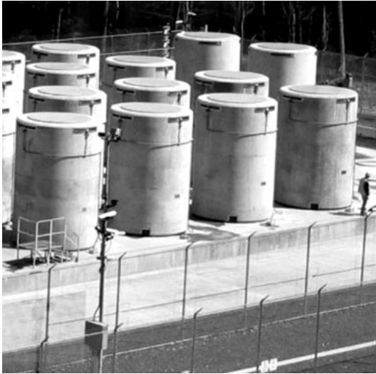
Figure 1.6: Dry cask storage at the Connecticut Yankee spent fuel storage facility. There are 43 dry storage casks on the site, of which 40 hold spent fuel and three store high-level radioactive waste. Source: Connecticut Yankee Atomic Power Company.
