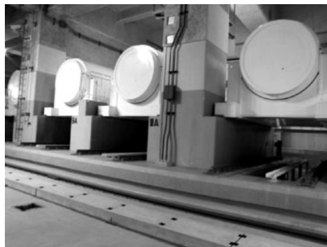
Figure 5.3: Dry metal cask storage facility at the Fukushima Daiichi nuclear power plant (left) and at the Tokai Daini nuclear power plant (right). The
