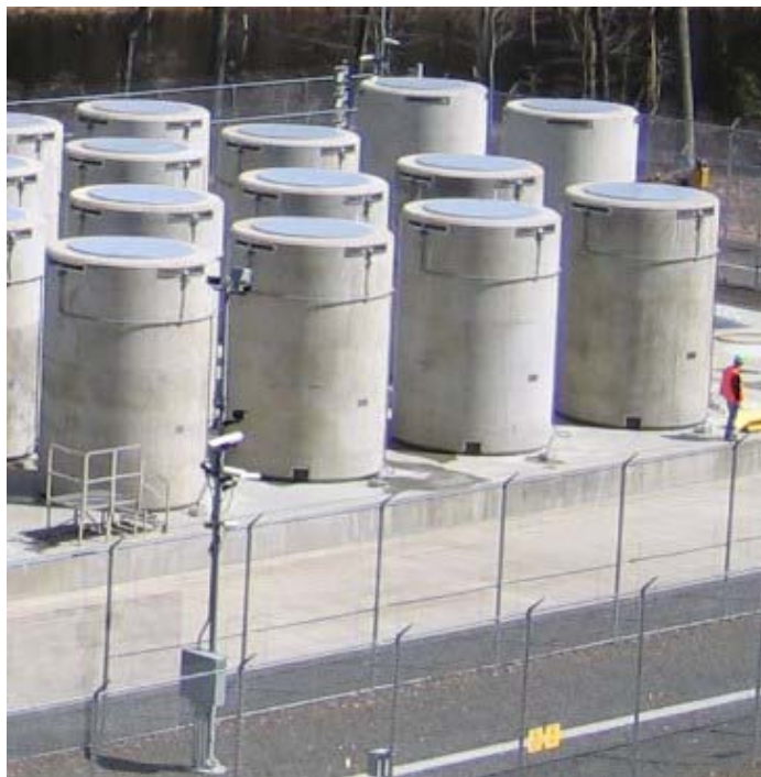
Figure 3. Dry cask storage at the Connecticut Yankee spent fuel storage facility. There are 43 dry storage casks on the site, of which 40 hold spent fuel and three store high-level radioactive waste. Source: Connecticut Yankee Atomic Power Company
