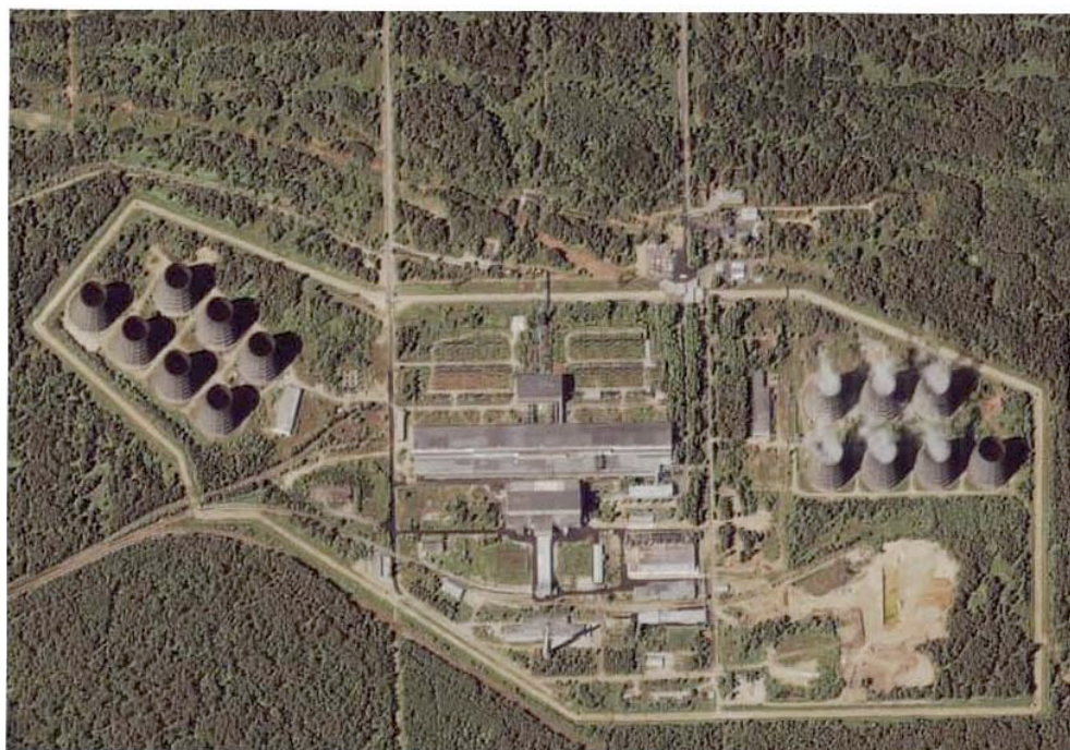
Figure 2. ADE 4 and 5 reactors, Seversk, July 10, 2000. The large building at the center is the turbogenerator building. The smaller building just below it houses the two reactors, of which only one was operating.
