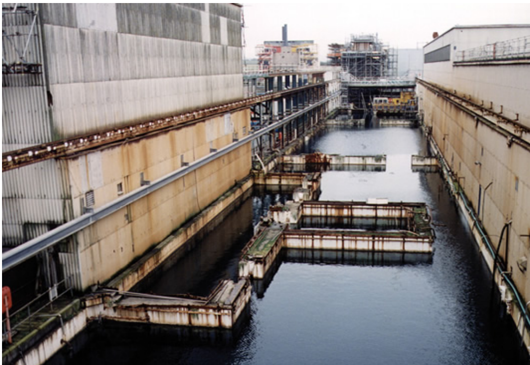
Figure 10. Magnox Fuel Storage Pond
