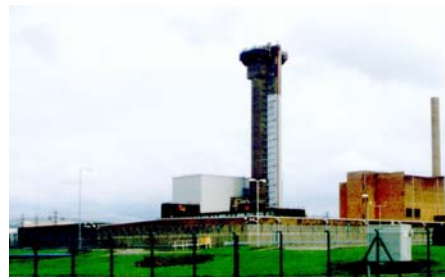
Remaining Pile No.1 Stack
