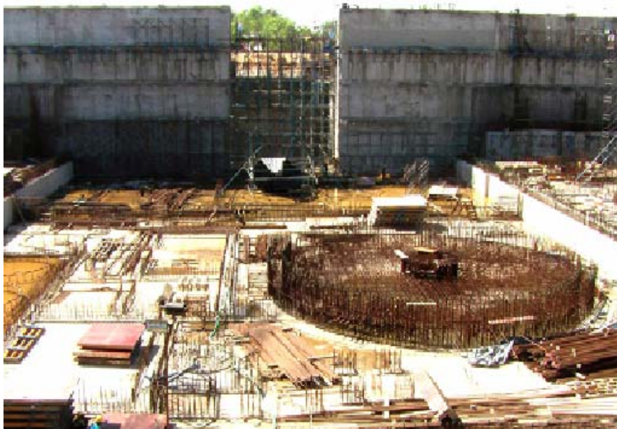
Figure 9. Construction activity at Prototype Fast Breeder Reactor, Kalpakkam, April 2006. 103
