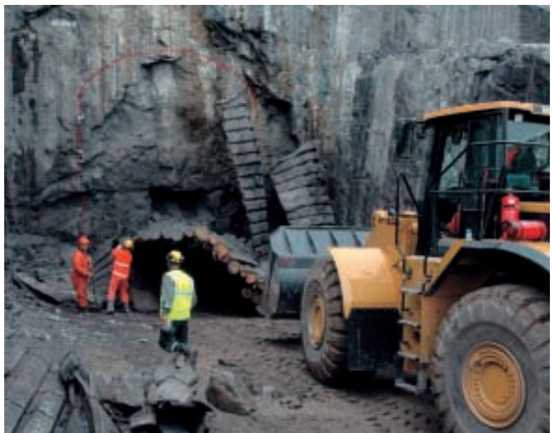
Blast signifying the start of work on the tunnel in September 2004
