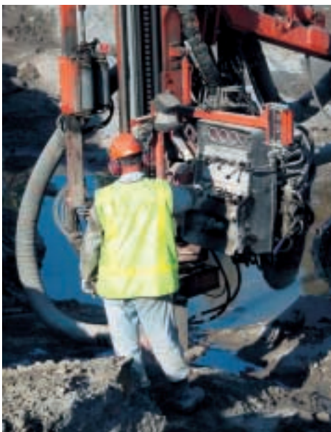
Excavation in June 2004
