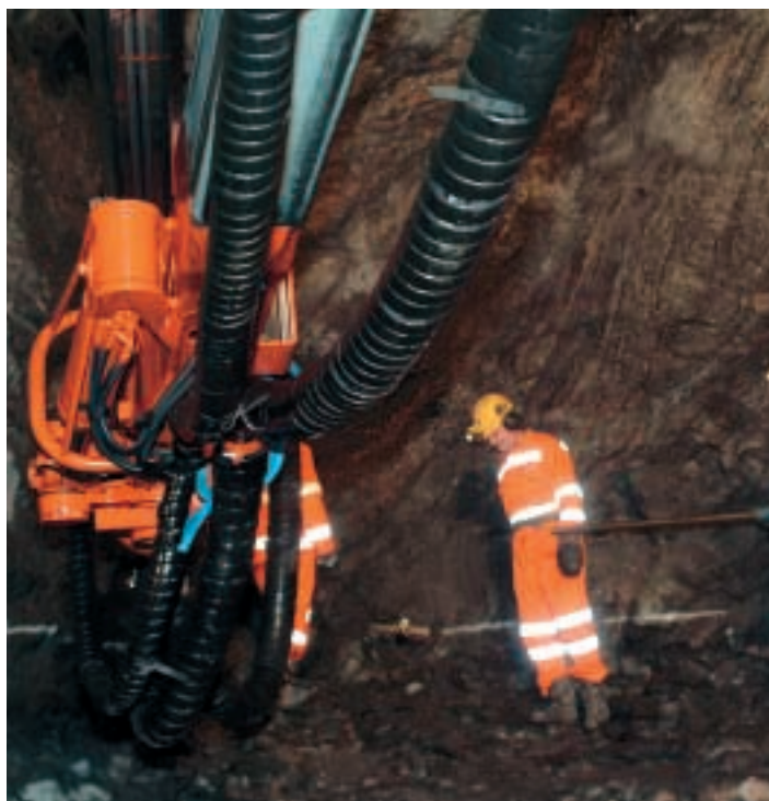
Drilling of grout holes
