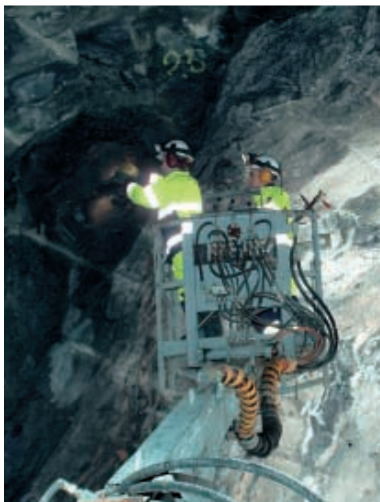
Map of the tunnel rock surface
