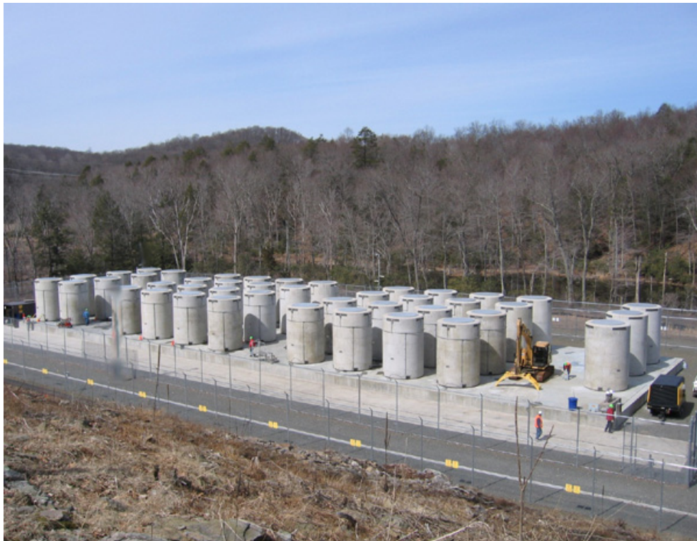
Figure 4. All the spent fuel (412 tons) discharged by the U.S. Connecticut Yankee Reactor (528 MWe), which operated from 1968 to 1998, is stored in 43 casks. The nuclear power plant itself has been completely removed and its site has been made available for other uses. 39
