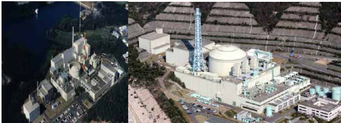
Figure 10. Japan's two breeder reactors. Left: The Joyo Experimental Fast Reactor (140 MWt) located in Oarai, near Tokai, began operations in 1978 and was shut down by a refueling accident in 2007. Right: The Monju sodium-cooled Prototype Fast Breeder Reactor at Tsuruga, Fukui Prefecture (280 MWe) was only connected to the grid from 29 August until 8 December 1995, when it had a sodium fire. Preparations for resumed operations in 2010 were terminated by a refueling accident. 86 Recently, preparations to restart Monju were halted again by the Nuclear Regulation Authority because of concerns about its safety management system. 87
