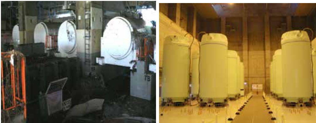
Figures 3 Left: Carbon steel spent fuel storage casks at the Fukushima Daiichi nuclear power plant after the tsunami had washed through the building. 34 Right: Dry cask storage at Tokai Daini nuclear power plant. 35 Each cask is 5 to 6 meters long and contains about 10 tons of spent fuel.
