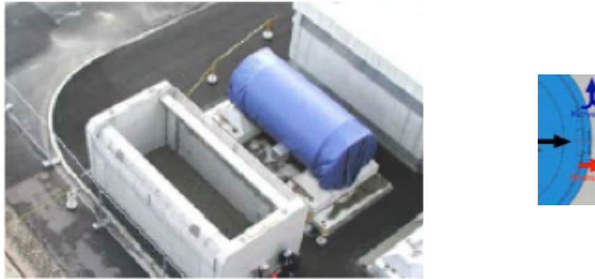
Figure 5. Left. Temporary protection for German storage casks pending construction of a permanent storage building. Right. The air around the casks is warmed by radioactive decay heat, rises and flows out of the slot at the top, and is replaced by cooler air entering through a slot at the bottom. 42
