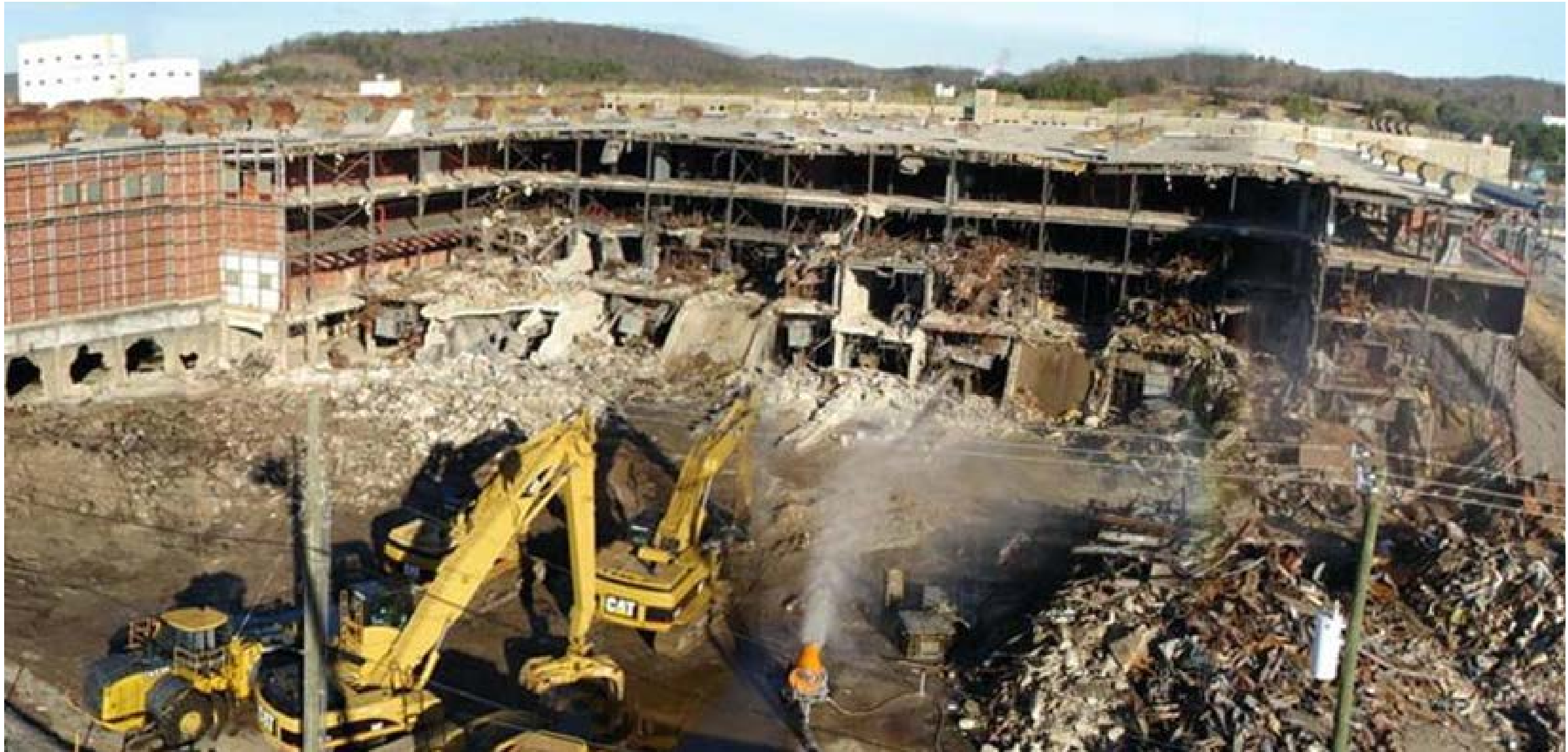
Demolition of first U.S. uranium enrichment plant in Oak Ridge, Tennessee
